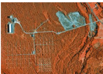
EISCAT Heating facility
